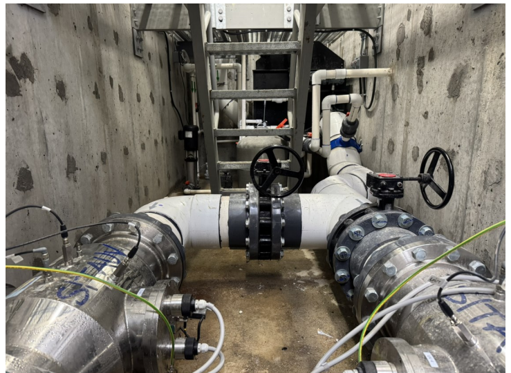
Effluent water filtration and UV disinfection in the basement of the water treatment building prior to discharge to the river.
