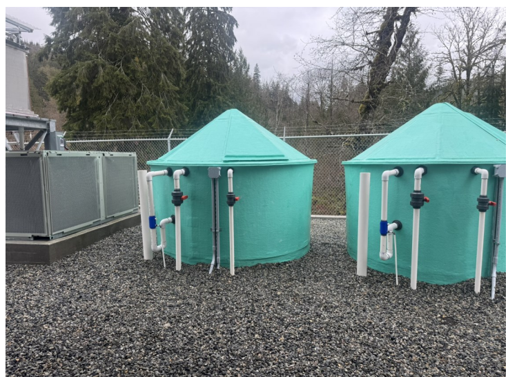
Broodstock holding tanks segregated at the back of the hatchery equipped with airlift recirculation to chill water in Summer.
