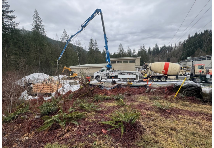
Pouring concrete in January 2024 for the water treatment trailer basement.
