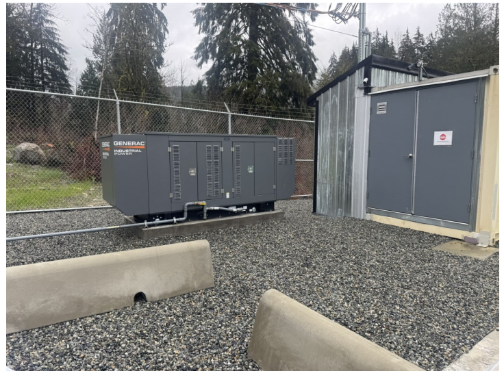
Backup power is provided by a 100 kW generator running off of propane fuel.
