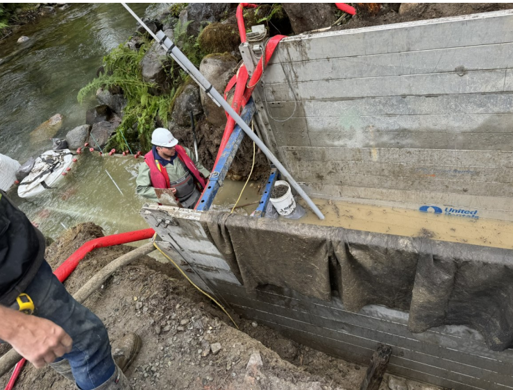
River intake construction during the least impact fisheries window was a constant effort of managing water in the excavation.
