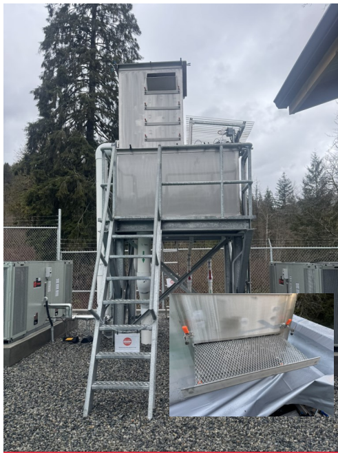
Degassing tower removes gases in the water. Water cascades through screens (inset)
